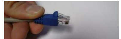
Slide boot back over lock clip
